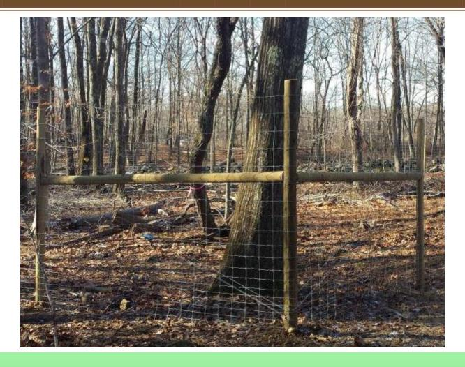
These pressure treated corner posts are reinforced with both horizontal posts and diagonally tensioned wire.
