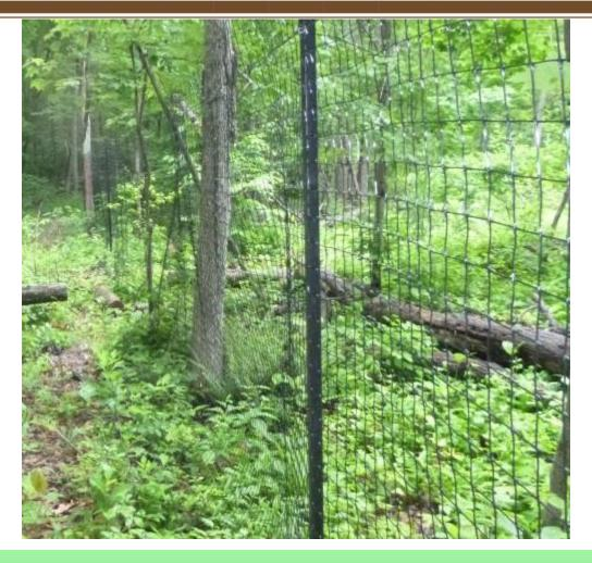
Metal posts are very strong, but can bend if hit by falling tree or branch. They are installed with a post pounder, meaning holes do not have to be dug. They cost \$10-\$15 each.
