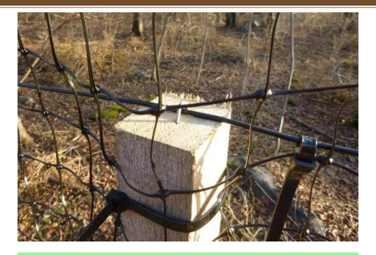
For wooden stakes, the guidewire can be attached to the top with a staple. The fence is then ziptied to the guidewire, and also to the stake. Zip ties also work great for attaching to metal posts.
