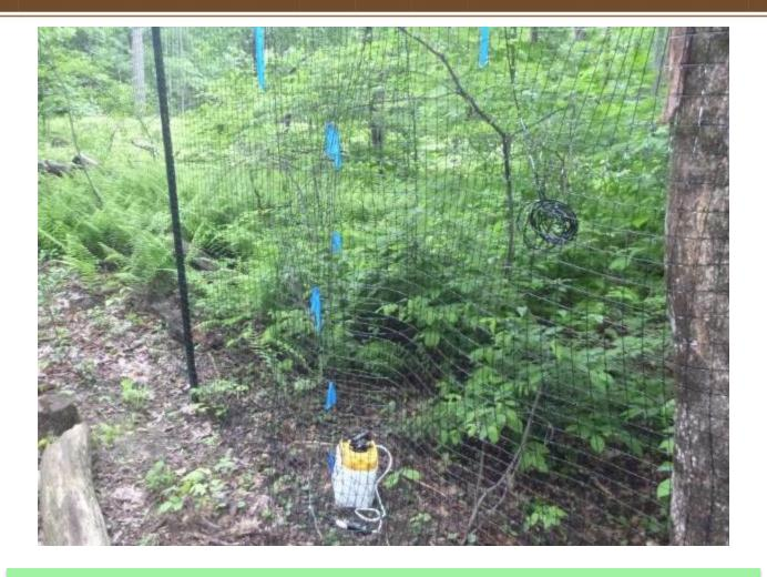
If you don't want to install a gate, basic entrance can be created by overlapping two fence sections and then holding them together with zipties or carabiners. This fence was flagged to make it visible from a distance
