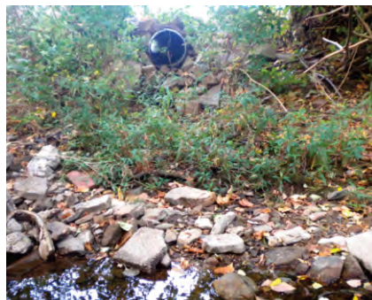
Drainage water delivered to a creek by pipe should have riprap protection around it and, if possible, should have to run through riparian vegetation before entering a stream.
